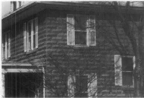
Illus. 3. Casting concrete to represent quarried stone was a popular late 19th-century technique seen in this circa 1910 mail-order house. While most components were delivered by rail, the foundations and exterior masonry were completed by local craftsmen. Photo: Sharon C. Park, AIA.
