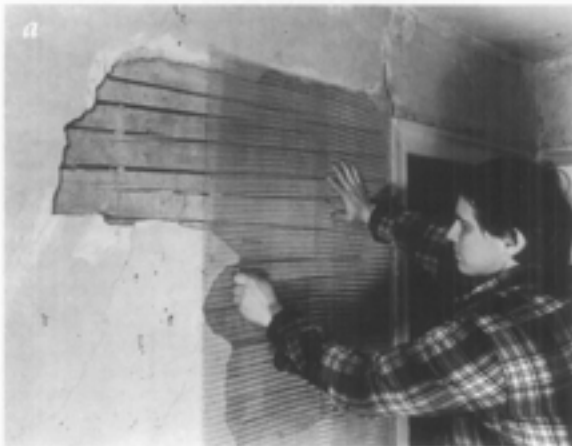
Fig. 10 (a) and (b). In this New Hampshire residence dating from the 1790s, the original plaster was a single coat of lime, sand, and horsehair applied over split lath. A one-coat repair, in this case, is appropriate. To the left: a flat sheet of galvanized expanded metal lath is placed over the patch area and an outline marked with a large soft lumber crayon. The metal lath is then cut to fit the hole and nailed to the lath. To the right: the edges of the original plaster and wood lath beneath have been thoroughly soaked with water. A steel trowel is used to apply the plaster in large, rough strokes. Finally, it will be scraped and smoothed off. Because only one coat of plaster is used, without a finish coat, a clean butt-joint is made with the original plaster. Photos: John Leek.
