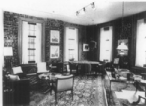
Figure 10. In this case plaster has been removed from perimeter walls, leaving brick exposed. In removing finishes from historic masonry walls, not only is there a loss of historic finish, but raw, unfinished walls are exposed, giving the interior an appearance it never had. Here, the exposed brick is of poor quality and the mortar joints are wide and badly struck. Plaster should have been retained and repaired, as necessary.
