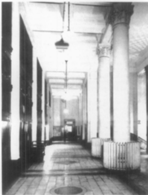
Figure 9. The tangible reminders of early mechanical systems can be worth saving. In this example, in the Old Post Office in Washington, D.C., radiators encircle Corinthian columns in a decorative manner. Note, too, the period light fixtures. These features were retained when the building was rehabilitated as retail and office space. Photo: Historic American Buildings Survey
