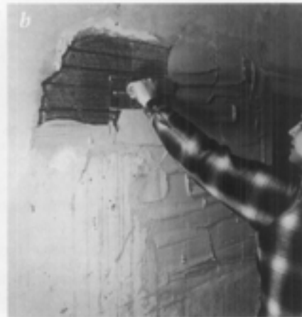
Fig. 10 (a) and (b). In this New Hampshire residence dating from the 1790s, the original plaster was a single coat of lime, sand, and horsehair applied over split lath. A one-coat repair, in this case, is appropriate. To the left: a flat sheet of galvanized expanded metal lath is placed over the patch area and an outline marked with a large soft lumber crayon. The metal lath is then cut to fit the hole and nailed to the lath. To the right: the edges of the original plaster and wood lath beneath have been thoroughly soaked with water. A steel trowel is used to apply the plaster in large, rough strokes. Finally, it will be scraped and smoothed off. Because only one coat of plaster is used, without a finish coat, a clean butt-joint is made with the original plaster. Photos: John Leek.
