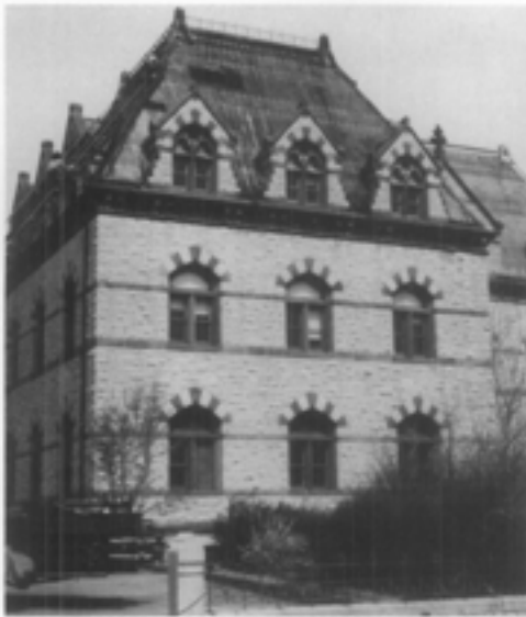
Overall Visual Character: Roof and Related Features
