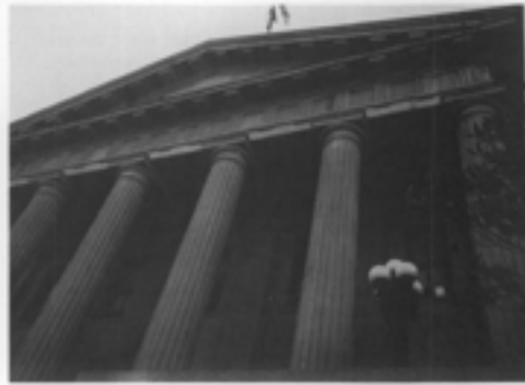
Illus. 13. Code-related changes are of concern in historic preservation projects because the integrity of the historic resource may be irretrievably affected. In the case of the Old San Francisco Mint, the fiberglass cornice was used to bring the building into seismic conformance. The original cornice was deteriorated, and the replacement (1982) was limited to the projecting pediment. The historic stone fascia was retained as were the stone columns. The limited replacement of deteriorated material did not jeopardize the integrity of the building. Photo: Walter M. Sonthheimer.
