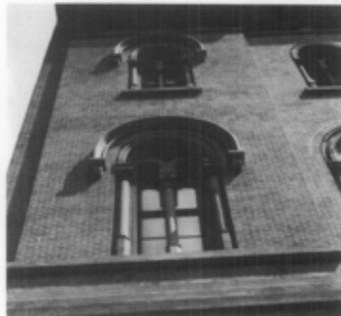
Illus. 8. Even when materials are not locally available, it may be possible and cost effective to find sources elsewhere. For example, the local sandstone was no longer available for the restoration of the New York Shakespeare Festival Public Theater. The deteriorated sandstone window hoods, were replaced with stone from Germany that closely matched the color and texture of the historic sandstone. Photo: John G. Waite.
