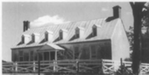
Overall Visual Character: Roof and Related Features
