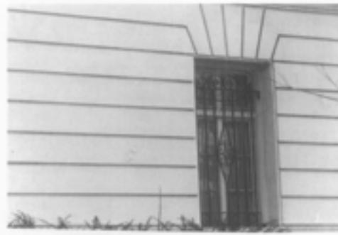
Illus. 2. Stucco has for many centuries represented a number of building materials. Seen here is the ground floor of a Beaux Arts mansion, circa 1900, which represents a finely laid stone foundation wall executed in scored stucco. Photo: Sharon C. Park, AIA.
