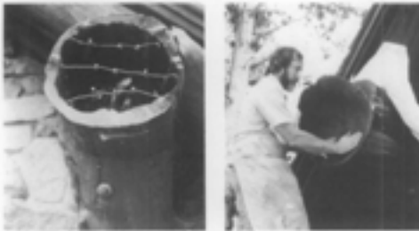
Illus. 17. Care must be taken to ensure that the replacement materials will work within a pre-designed system. At the Norris Museum, Yellowstone National Park, the 12-inch diameter log rafters, part of an intricate truss system, had rotted at the inner core from the exposed ends back to a depth of 48 inches. The exterior wooden shells remained intact. Fiberglass rods (left photo) and specially formulated structural epoxy were used to fill the cleaned out cores and a cast epoxy wafer end with all the detail of the original wood graining was laminated onto the log end (right photo). This treatment preserved the original feature with a combination of repair and replacement using substitute materials as part of a well thought out system. Photos: Courtesy of Harrison Goodall.
