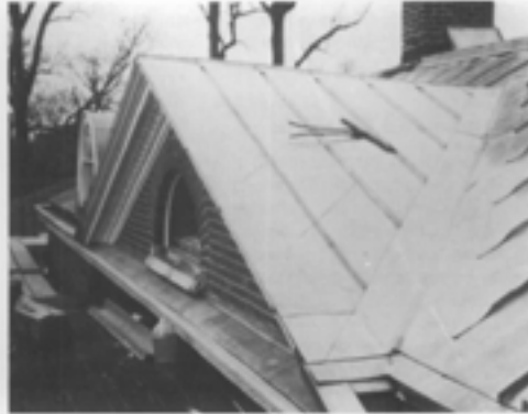
Illus. 12. Substitute materials may be considered when the original materials have not performed well. For example, early sheet metals used for roofing, such as tinplate, were reasonably durable, but the modern equivalent, terne-coated steel, is subject to corrosion once the thin tin plating is damaged. Terne-coated stainless steel or lead-coated copper (shown here) are now used as substitutes. Photo: John G. Waite.
