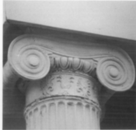
This replica column capital was made using epoxy resins poured into a mold taken from the building. The historic wooden column shaft was repaired during the restoration. Photo: Courtesy Dell Corporation.
