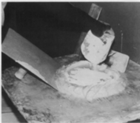
Fig. 17. This contemporary plasterer is mixing a lime finish coat in much the same way as America's earlier artisans. The ring consists of lime putty; the white powder inside is gauging plaster. After the mixture is blended, a steel trowel will be used to apply it. It should be noted that a traditional lime finish coat can be applied over a veneer plaster base coat to approximate the look of historic plaster walls and ceilings. Photo: Marylor MacDonald.
