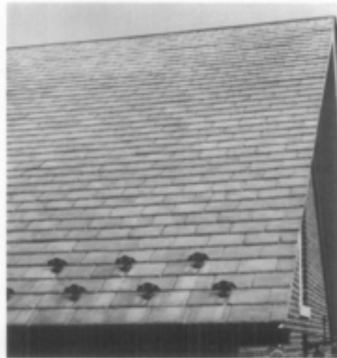
Illus. 14. The visual qualities of the historic feature must be matched when using substitute materials. In this illustration, the lighter weight mineral fiber cement shingles used to replace the deteriorated historic slate roof were detailed to match the color, size, shape and pattern of the original roofing and the historic snow birds were reattached. Photo: Sharon C. Park, AIA.
