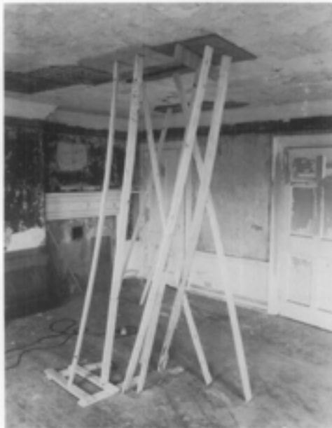
Fig. 15. When ceiling repairs are made with wet plaster or with an injected adhesive mixture, the old loose plaster must be supported with a plywood brace until re-keying is complete. Photo: John Leek.
