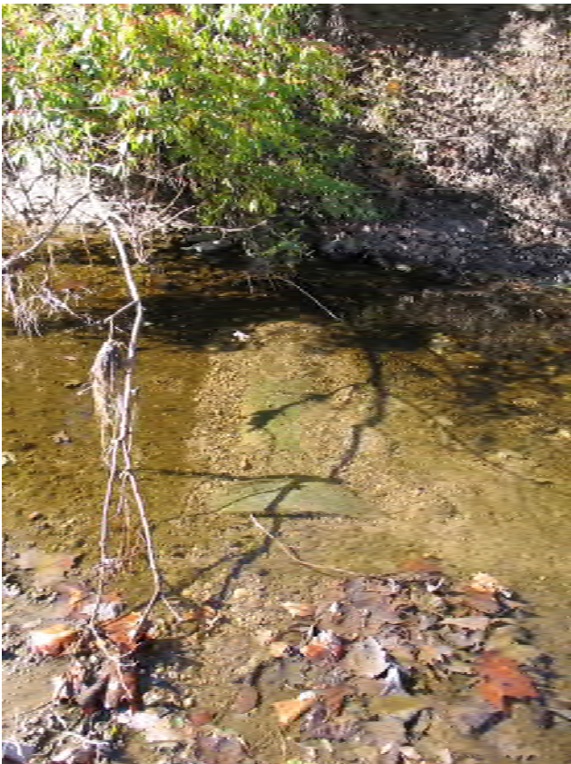
Existing trunk sewer pipe & joint exposed – west side creek bank
